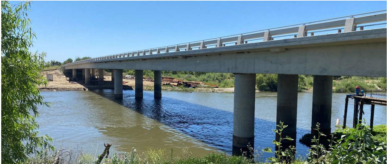
Photo of the new bridge structure.
