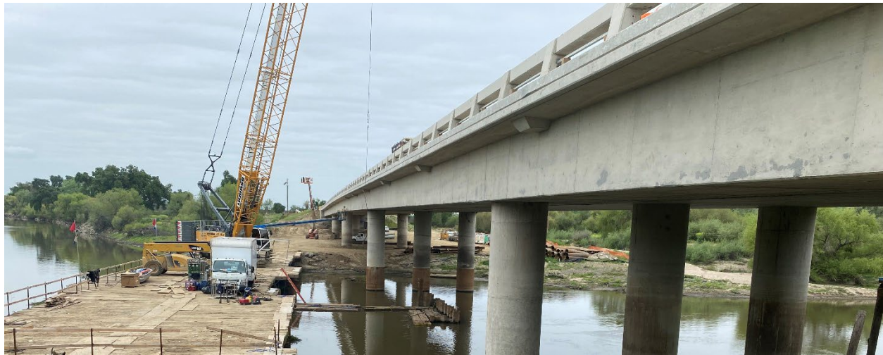
Photo of the new bridge structure and staging area.
