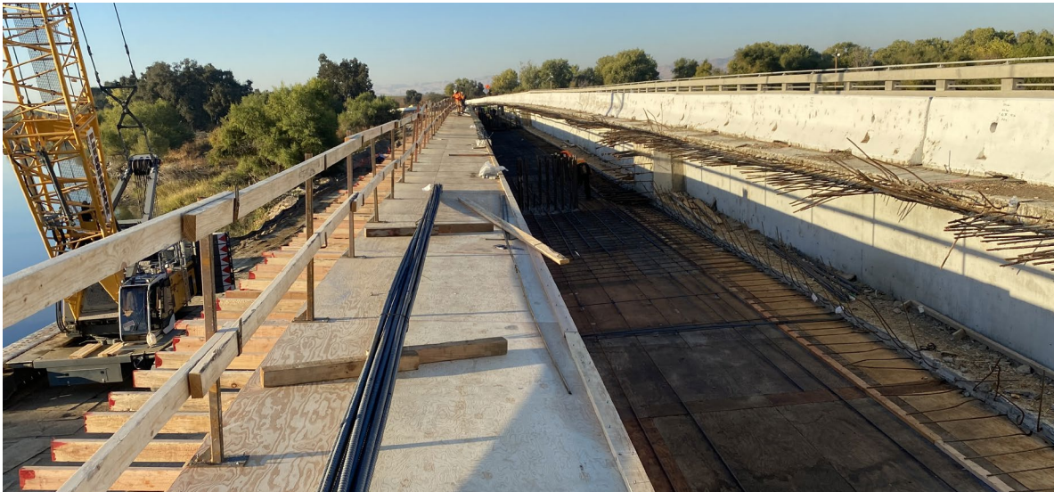
Photo of the new bridge superstructure.
