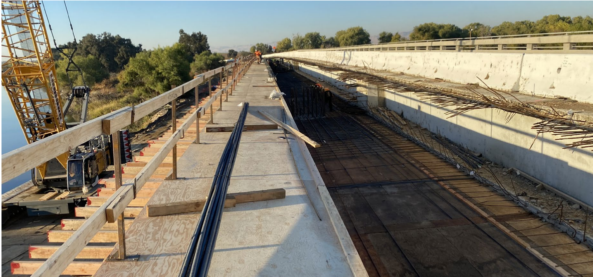
Photo of the new bridge superstructure.
