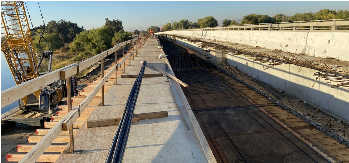
Photo of the new bridge superstructure.
