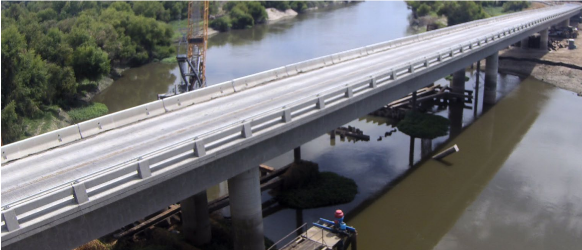
Photo of the new bridge structure.
