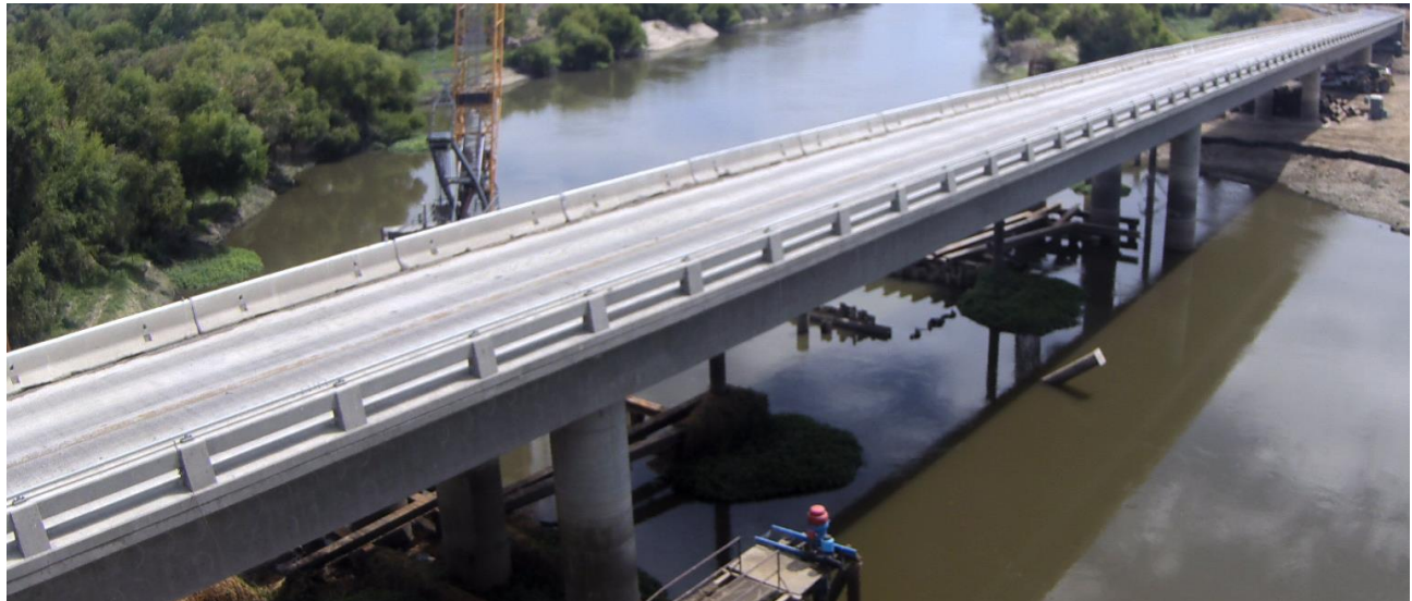
Photo of the new bridge structure.
