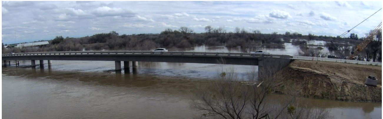
Photo of the new bridge structure looking from the north side.
