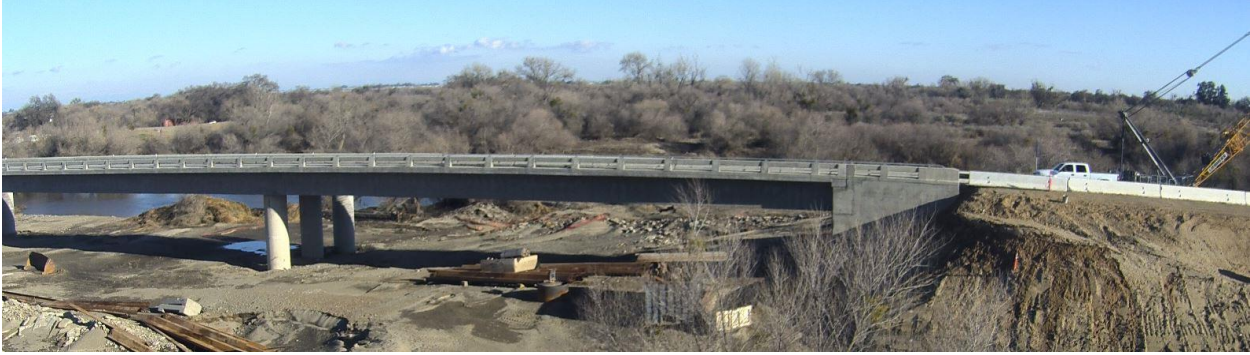
Photo of the new bridge structure looking from the north side.
