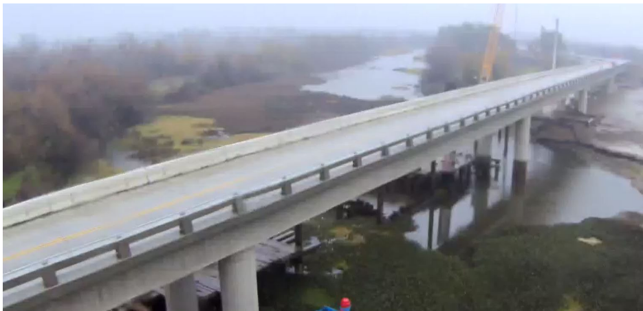
Photo of the new bridge structure looking south.
