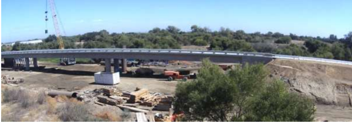
Photo of the new bridge structure looking from the north side of the new bridge.
