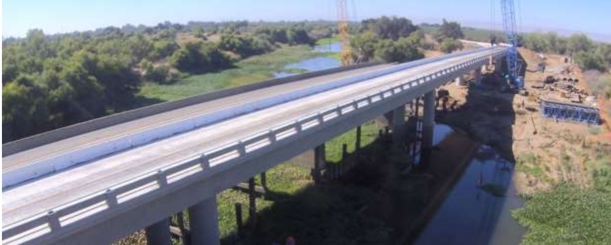
Photo of the new bridge structure looking south.
